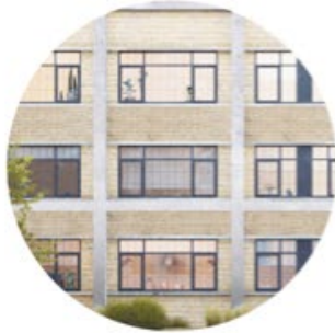
2. Proposed concrete structural frame
