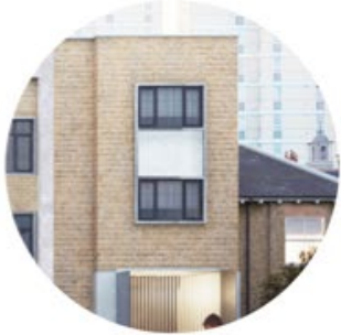
1. Existing concrete details around windows
