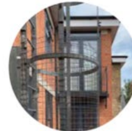
Metal Components Existing metal escape stairs
