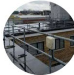
Metal Roofing Components Existing metal balustrades on roof
